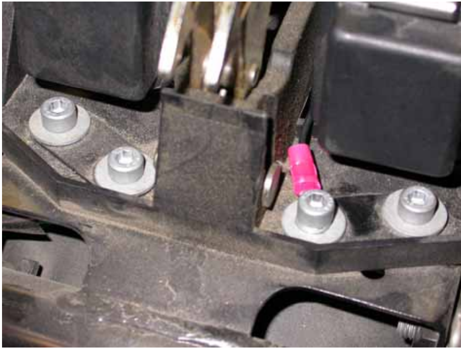
Figure 19. Ground wire connected
