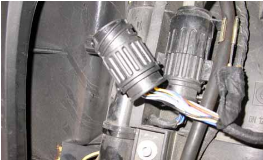
Figure 12. Wrapping cut back to expose the wires
