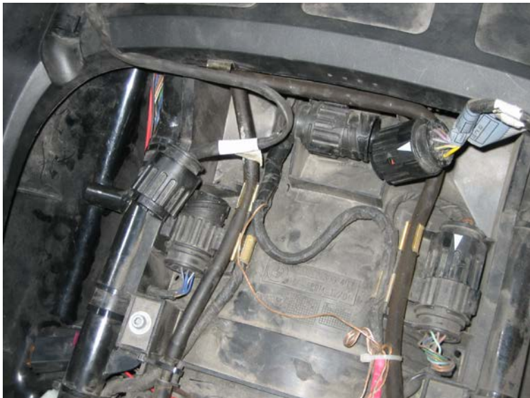
Figure 2: Two wiring harness connectors shown disconnected (pre-2005 model LT).
